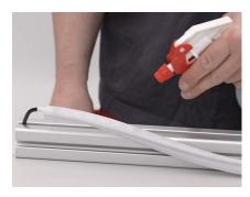
Before pressing in the casing profile with the LED strip, dampen the Line 8 groove with a little soapy water.
